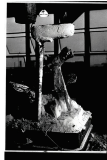
Pegasus being removed from the mold
